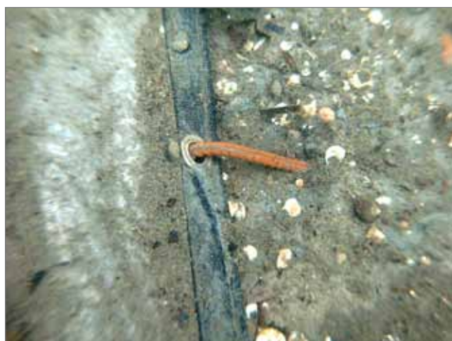
Figure 10. Iron reinforcing rods were used to secure the edges of the geotextile. Photo Staffan von Arbin, Bohusläns museum.
