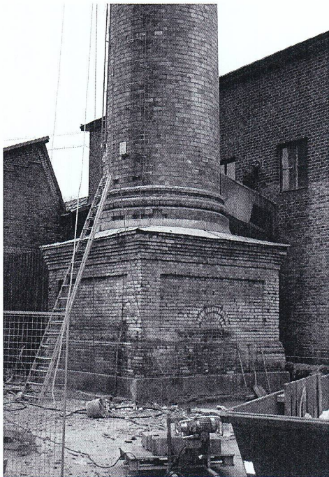
Fundamentet under restaurering.
